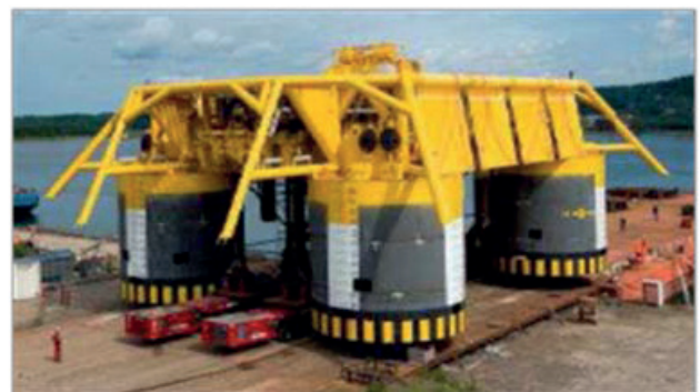
Figure 4.9. Template with skirted foundation at Ormen Lange (Neerland, 2006).
